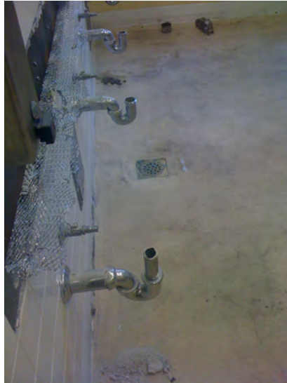
Bathroom sinks being lowered
